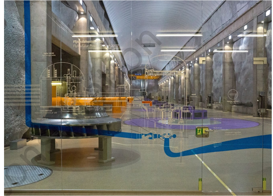
Photo 70: Inside Fljotsdalur power station, machine hall in the background
