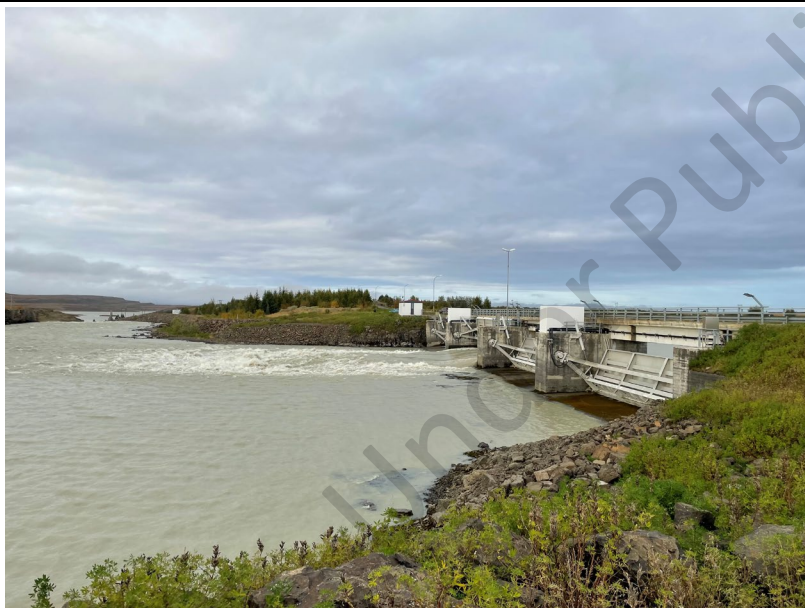
Photo 57: Lagarfoss Hydropower plant
