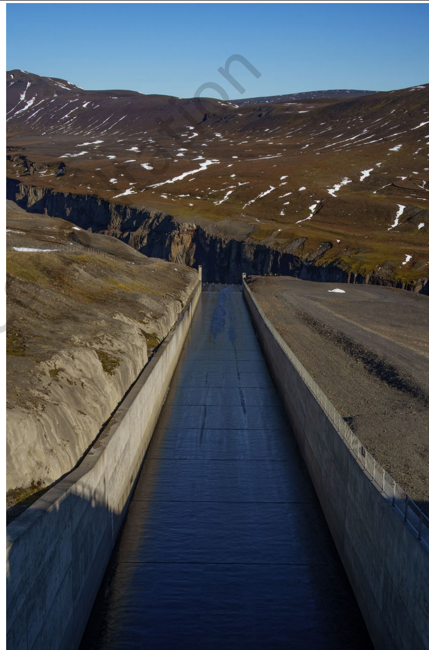
Photo 26: The spillway at the Kárahnjúkar Dam
