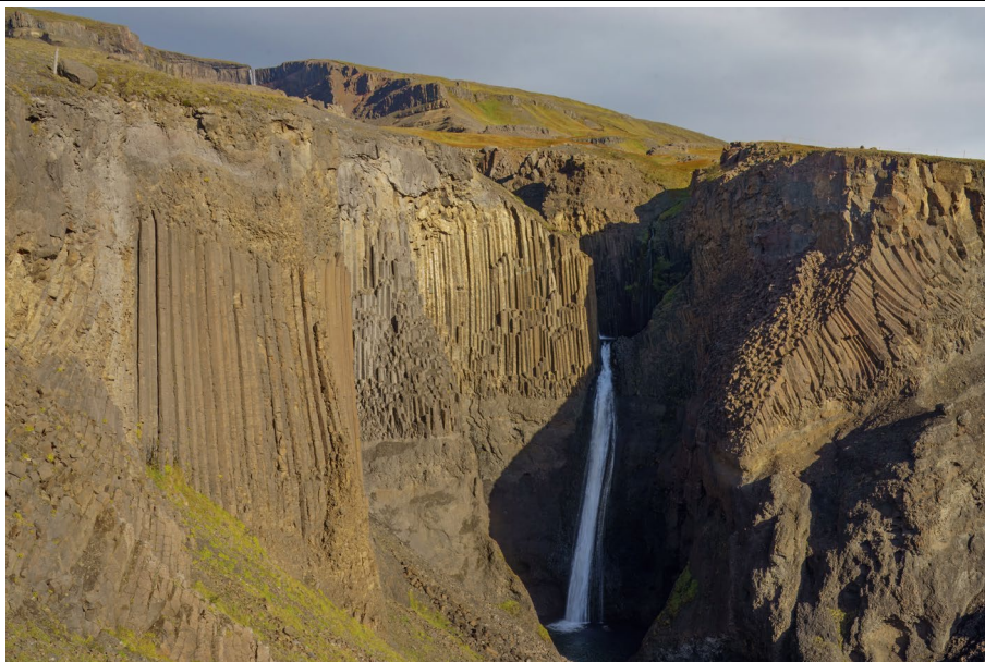
Photo 15: Litlanesfoss, near Fljótsdalsstöð power station
