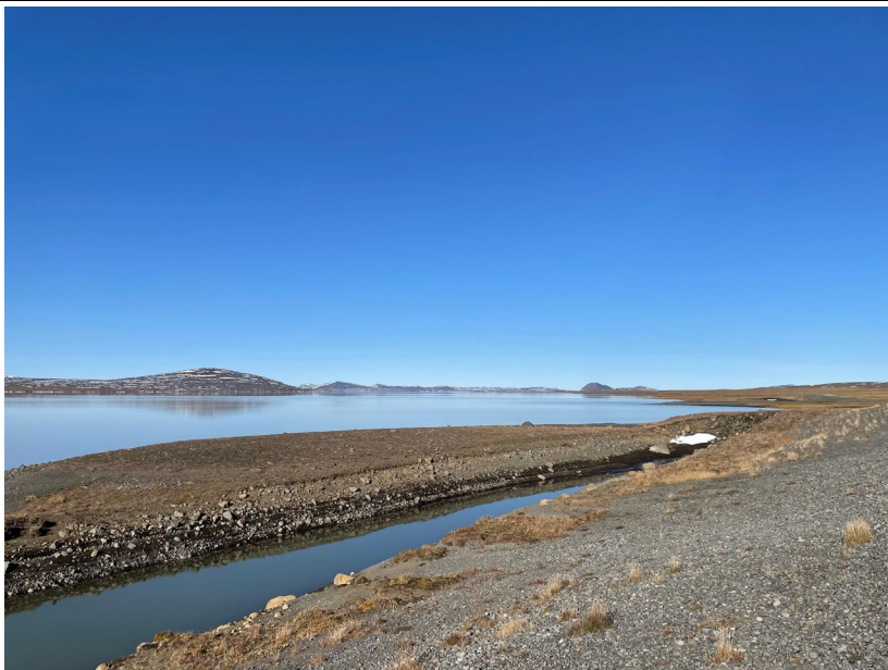
Photo 55: Sand traps along Kárahnjúkar Reservoir
