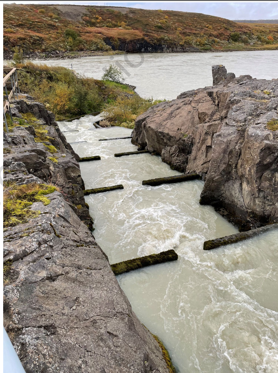
Photo 54: Fish ladder at Lagarfoss
