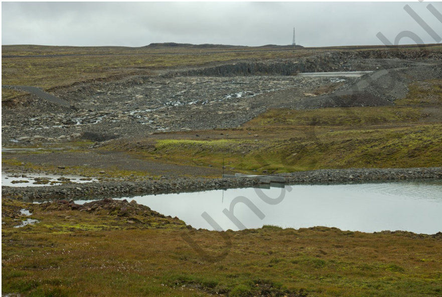
Photo 71: Kelduarlón spillway with dam-leakage monitoring in foreground
