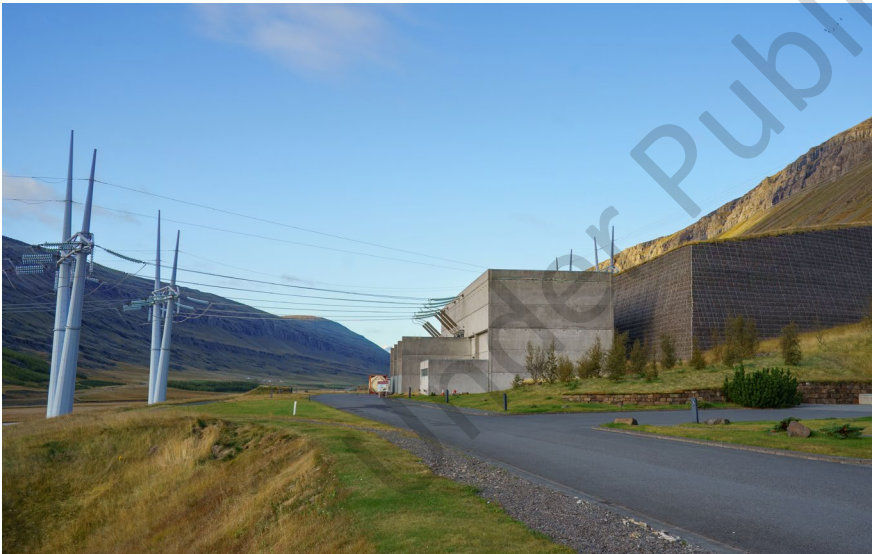
Photo 7: Fljótsdalsstöð power station
