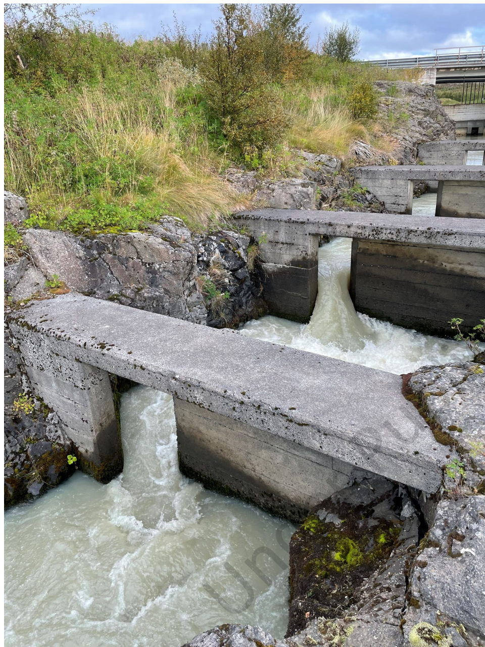
Photo 53: Fish ladder at Lagarfoss
