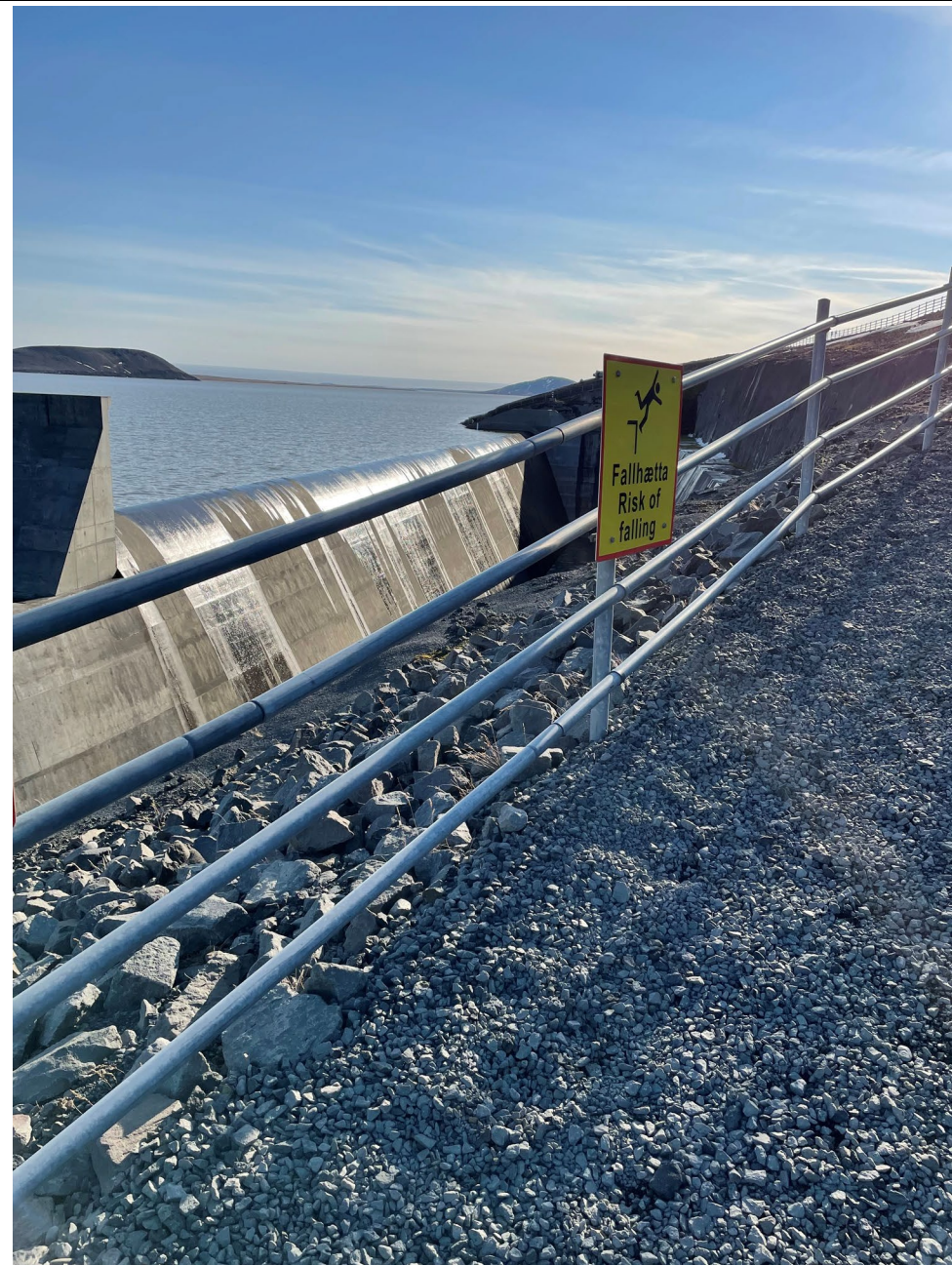
Photo 59: Safety signage at Kárahnjúkar Dam
