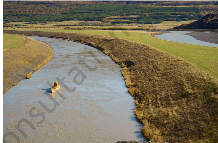
Photo 28: The tailrace canal below Fljótsdalsstöð power station with boat art work in the canal
